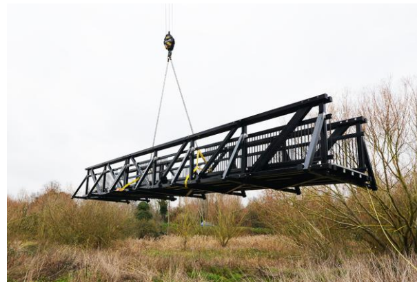
Steel bridleway bridge, large span ~£150k +
