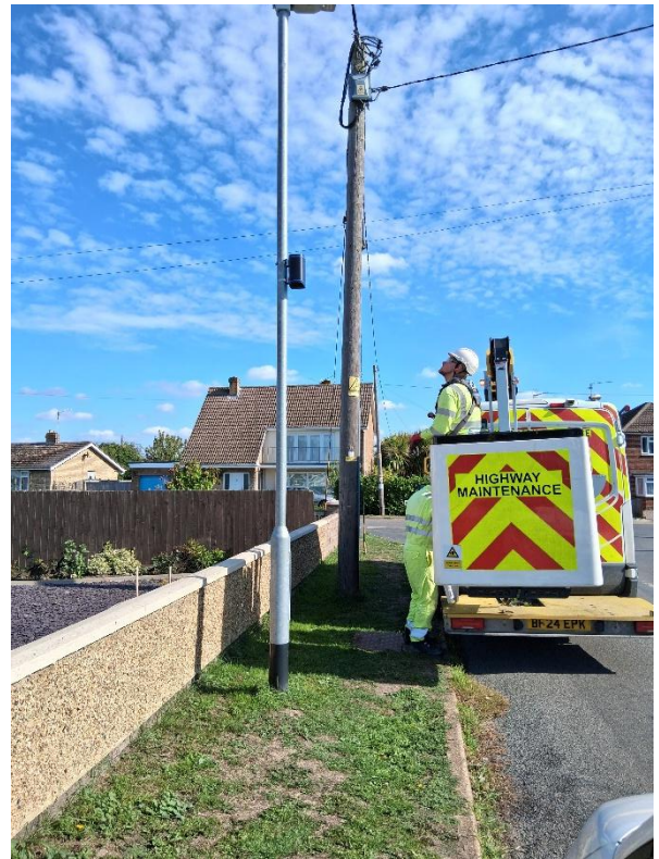
Right: Zephyr and solar panel installed
