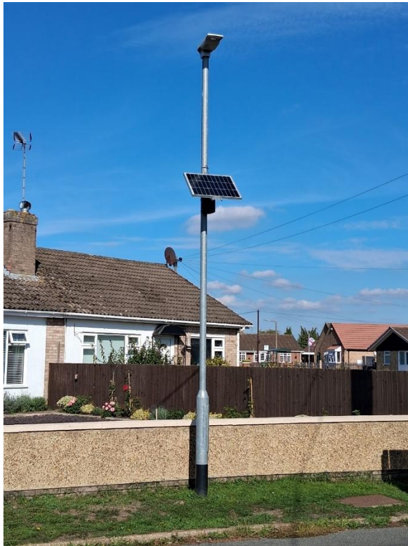
Left: Zephyr during installation
