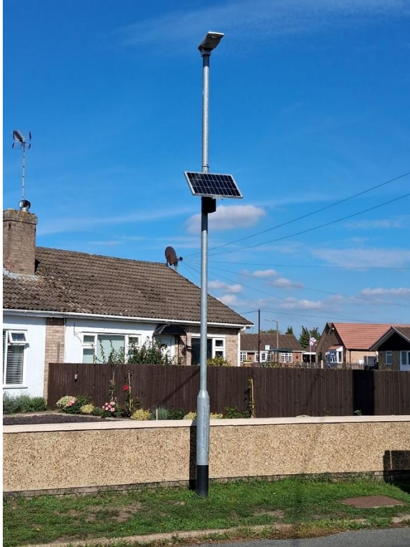
Left: Zephyr during installation
