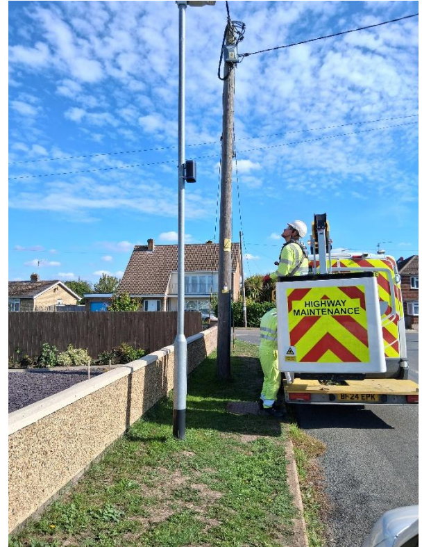
Right: Zephyr and solar panel installed
